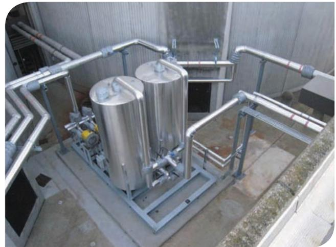
*The cogeneration system project included the installation of a new gas conditioning unit.*
