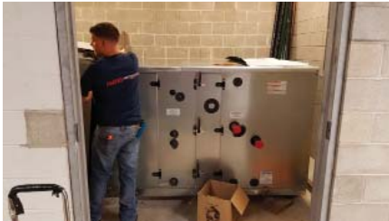
Installation of New Air Handling Units
