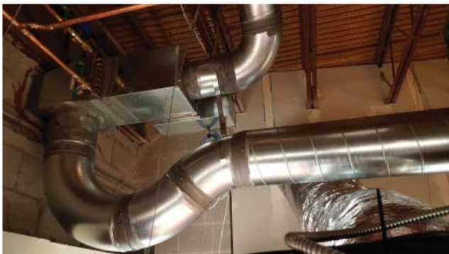
New Variable Air Volume Unit
