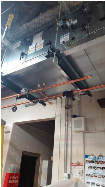
Installation of New Air Handling Units
